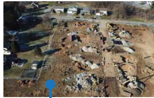
Buildings are razed for construction
