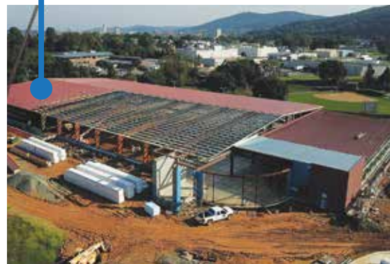
Roof nearly completed
