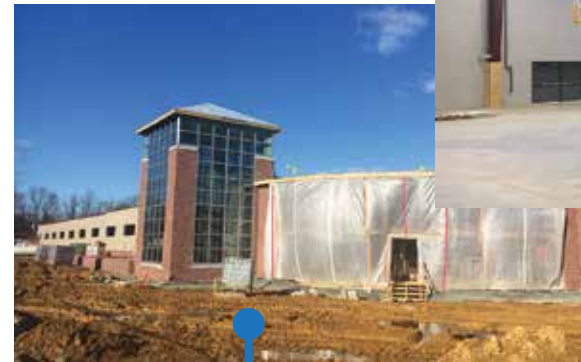
Walls go up
