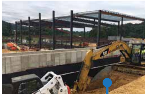
Structure beams go up
